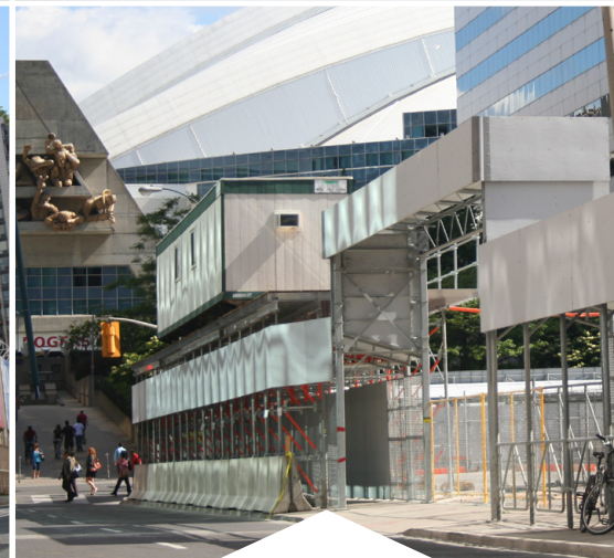
Covered Walkway with Office Trailer Support
